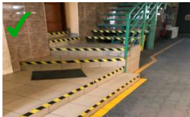
Figure 85: Steps and stairs properly marked to avoid falls
