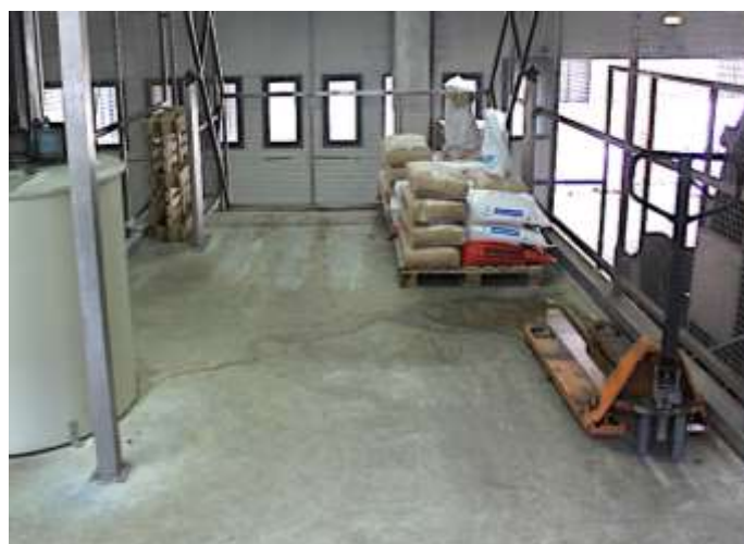
Figure 22: Correct flooring for transporting chemicals around the workplace
