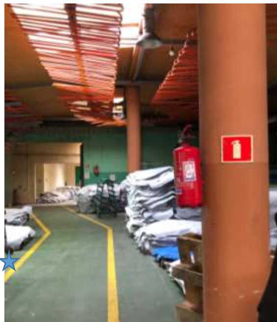
Figure 138: Keep evacuation routes unobstructed and fire fighting equipment ready in marked locations
