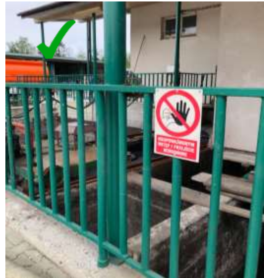
Figure 98: Restricted access to confined spaces within ETP:
