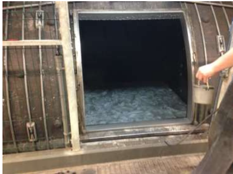
Figure 139: H 2 S can accumulate in drums and make operators fall inside when taking samples. Be prepared for this!
