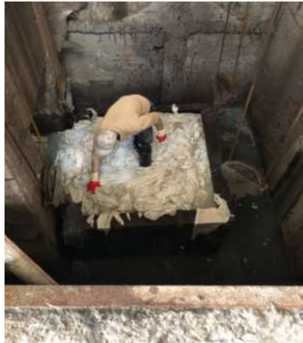
Figure 96: Unprotected man performing a task in confined space
