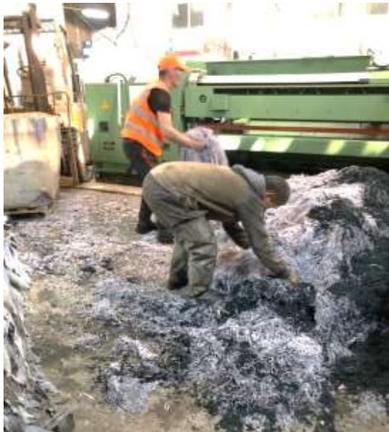
Figure 122: Removing shavings or other material manually is less effective and imposes direct contact with shavings
