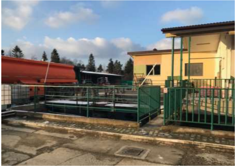
Figure 140: There are numerous confined spaces within ETPs. You need to take special care in guarding them and while cleaning and maintaining
